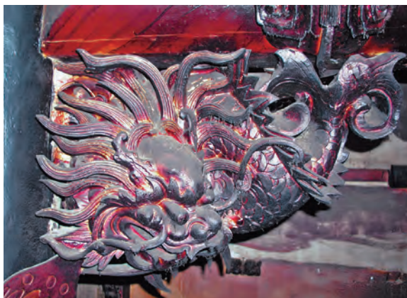
圖11. 正殿四點金柱鰲魚插角 Figure 11. Cha-Jiao carved as dragon-head fish in the a group of four golden pillars of the main hall
